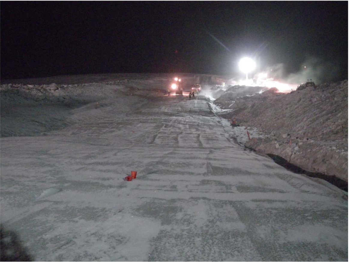
Photo 12 Cleaning of key trench looking SW along trench. Note snow starting to fall on nightshift.
