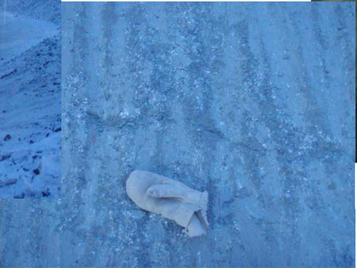
Photo 6: Close up view of surface around 1+50 where 5/8" removal is nearly complete. Note the faint line showing the approx.. location where overlying lift tapered out.
