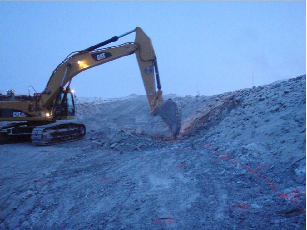
Photo 3: 345 excavator scraping 5/8" material cover from key trench around station 1+85
