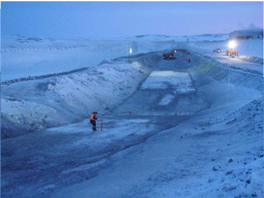
Photo 5: ~NE view down key trench. Note the whiter, frost covered, area in the center to eastern side of the picture shows the area where material on 2012/01/24 was placed.
