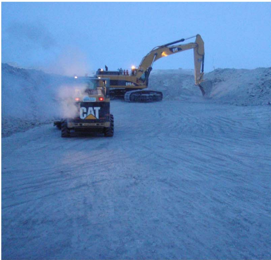
Photo 4: Bobcat with brush and 345 excavator cleaning key trench from ~ 1+40 to 1+85, ~NE view.
